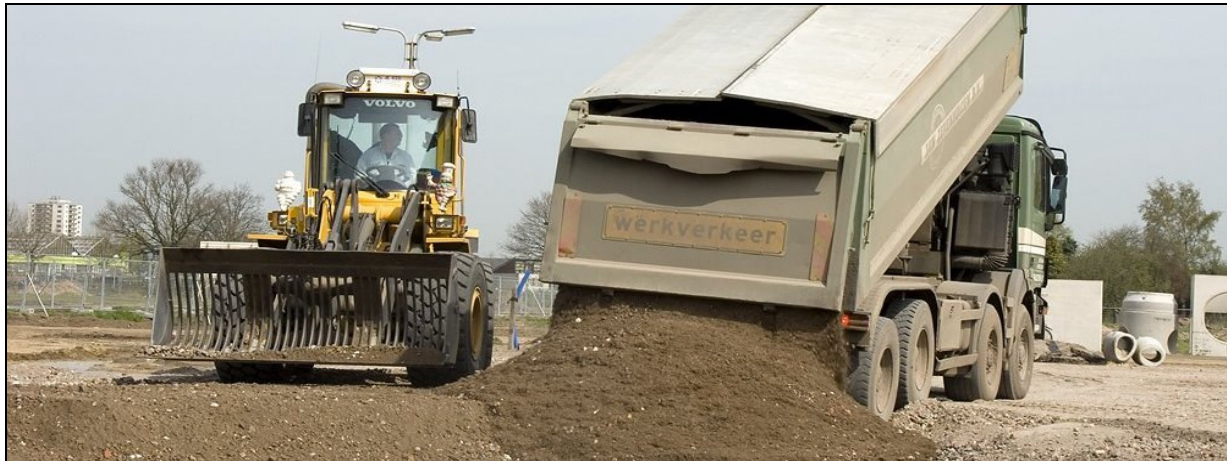
Figure 54: construction of an unpaved road.
