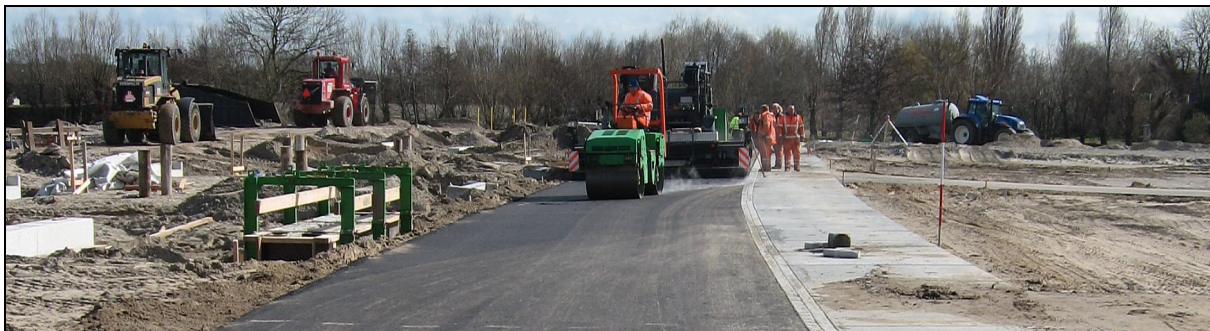
Figure 28: construction of temporary roads on Duyfrak.
