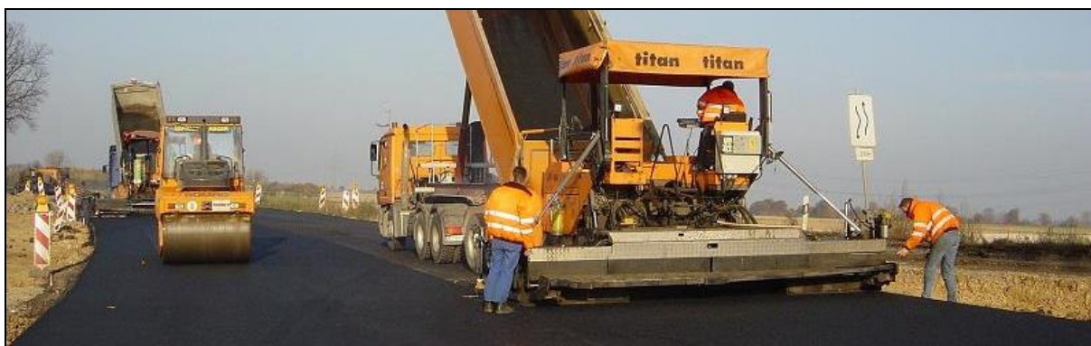
Figure 59: construction of an asphalt pavement.
